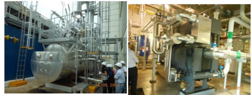
Heat recovery steam generator of tri-generation system (left) and absorption chiller
